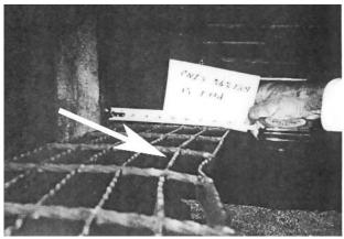
the railroad, YJB attorneys had performed an exhaustive investigation of the accident and had discovered, despite the railroad's best efforts to suppress the information, that this photo existed prior to modification to the car, which proved that the platform was bent and defective.
